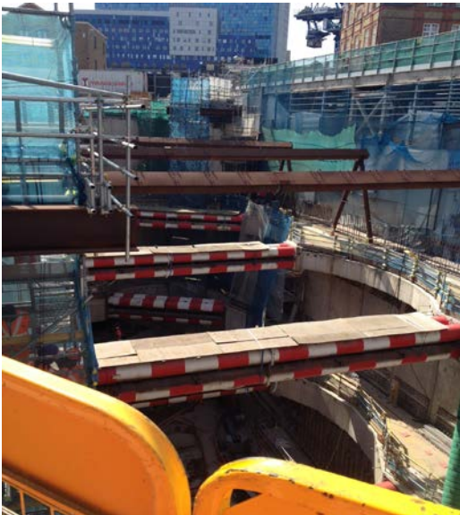
Whitechapel Station, Durward Street shaft under construction.
