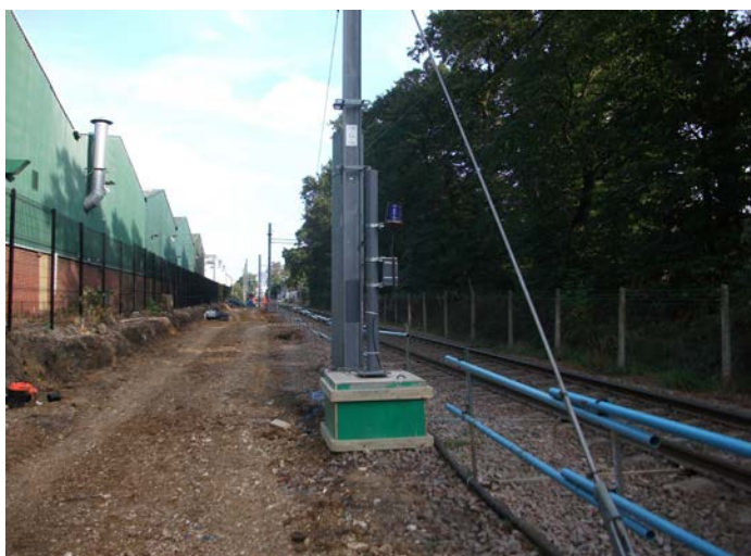
Twin tracking works
